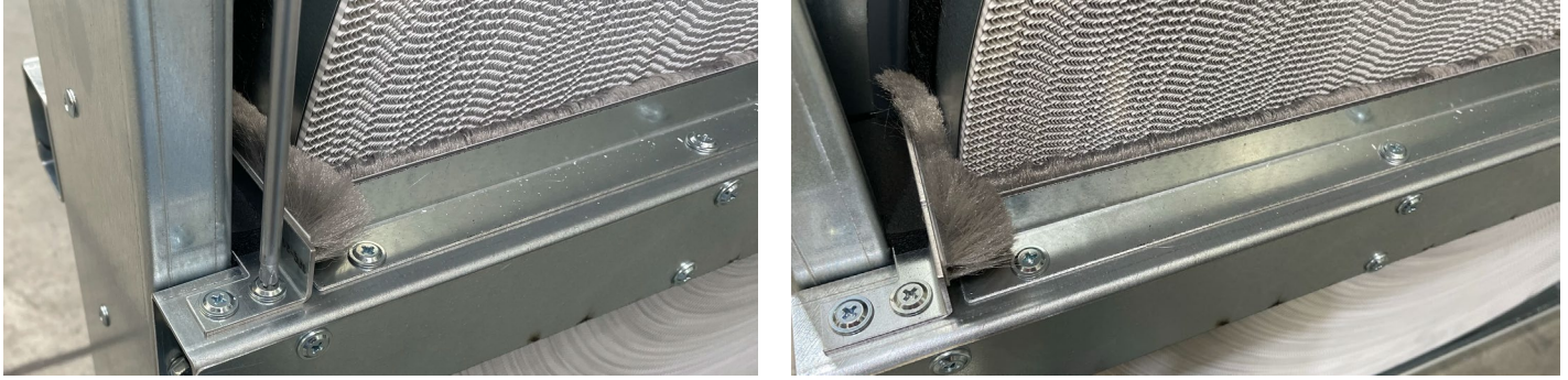
Figure 13 – Main Brush Rail installation
