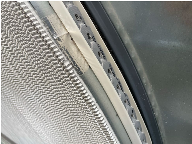
Figure 22 - Belt arrangement on the wheel and pulley
